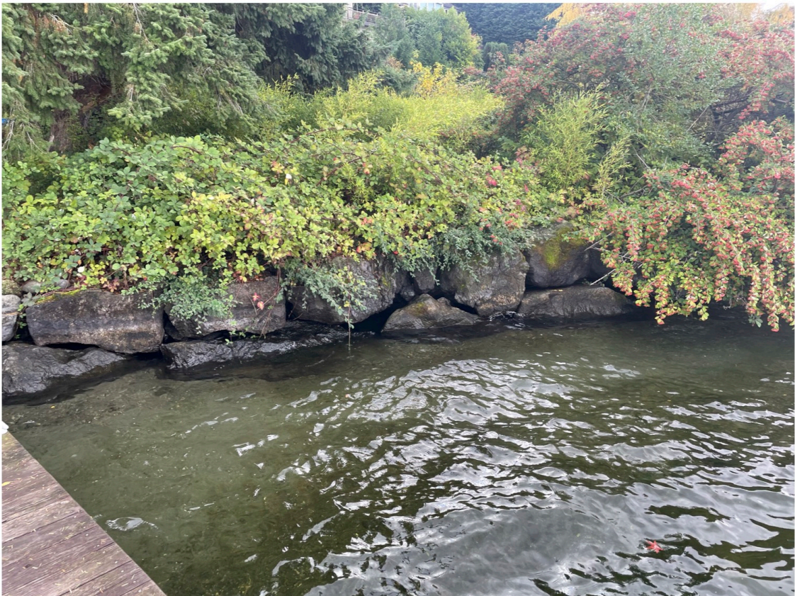
Photo 4 - Existing shoreline looking south.
