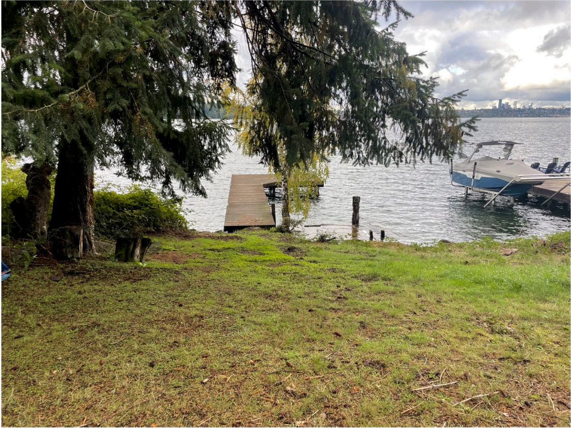
Photo 1 - Existing conditions looking waterward.
